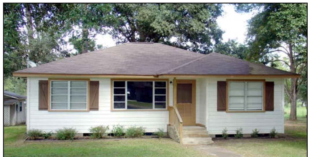
Hockley: Charming wood frame home on 1.285 acres in Magnolia ISD. Very clean, well-cared for home with hardwood & laminate floors, formals and cute country kitchen with white cabinets. New aerobic septic system, A/C, furnace & electric service in 2014. Nice 24x40 detached garage/shop with concrete floor. Beautiful park-like setting with lots of shade and fenced on all sides.....PENDING...$175,000
